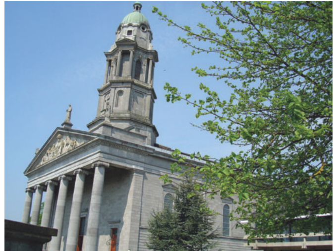
The renovation project at St Mel's Cathedral will create dozens of jobs in a town blighted by unemployment.
